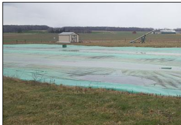
Manure storage with a cover and flare system
