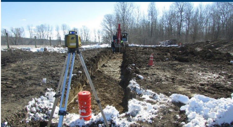
Left: Livingston County installation of underground outlet and water and water and sediment control basin.
