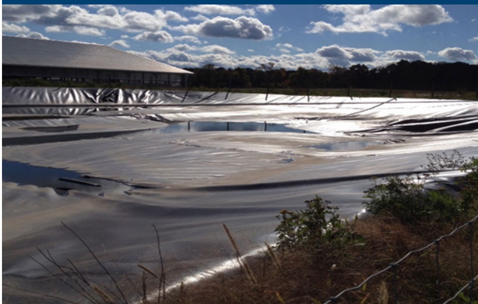
Impermeable cover on a manure storage to reduce methane emissions, eliminate rainwater from entering the storage, and reduce waste runoff into water bodies.
